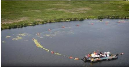
**We continue to make important progress with our multi-million-dollar effort to reduce flood risk along the Yahara Chain of Lakes.** Sediment removal that started in the river channel this summer is designed to improve flow, moving rainwater that currently sits in our lakes for weeks thru at a steadier clip. This year's work is focusing on the area between Lakes Monona and Waubesa and is
